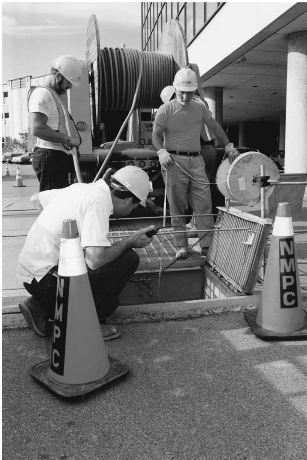
Figure 8-5 Installing cables.
