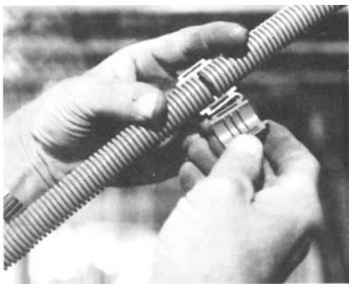
Figure 18-10 ENT quick-connect coupling. (Courtesy of Carlon Electrical Sciences, Inc.)
