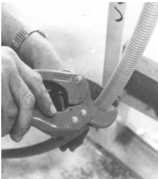
Figure 18-13 Cutting ENT. (Courtesy of Carlon Electrical Sciences, Inc.)
